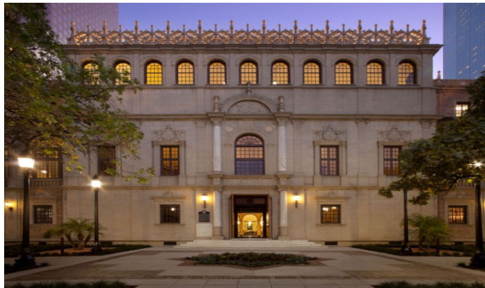
McKinney Entrance to the Julia Ideson Building, Photo by Joel Draut
